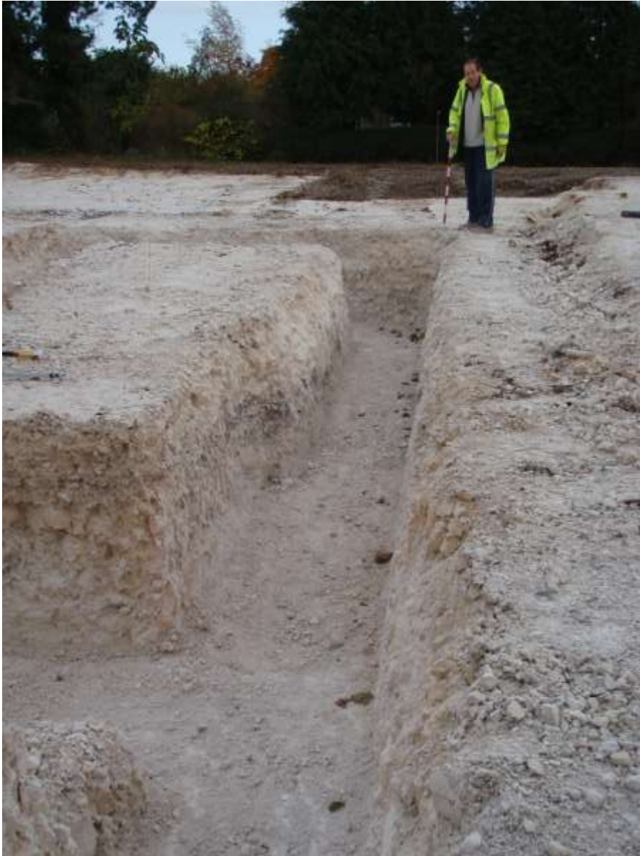
Plate 6. View of the trenches Plot 2 (looking NW)
