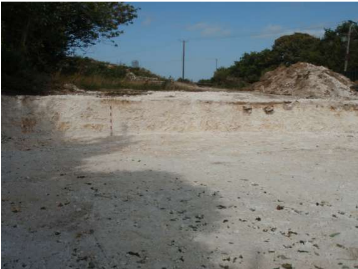
Plate 3. View of site reduction Plot 1 (looking N)
